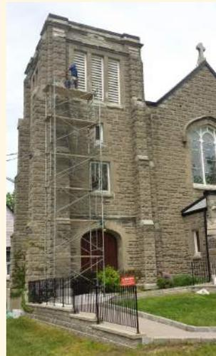
In January **1995** the church received a report from McNeely Engineering Consultants Ltd (Kingston). At that time, they identified significant deterioration of the tower, due to ongoing water penetration and seasonal freeze-thaw action. They recommended a comprehensive program of restoration, but no work was done to repair the tower exterior.
